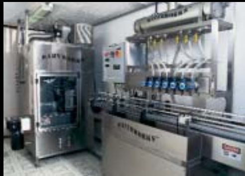
Custom Electrical, Plumbing, Insulation Installation
